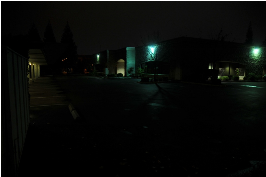
Existing 175 Watt MH
